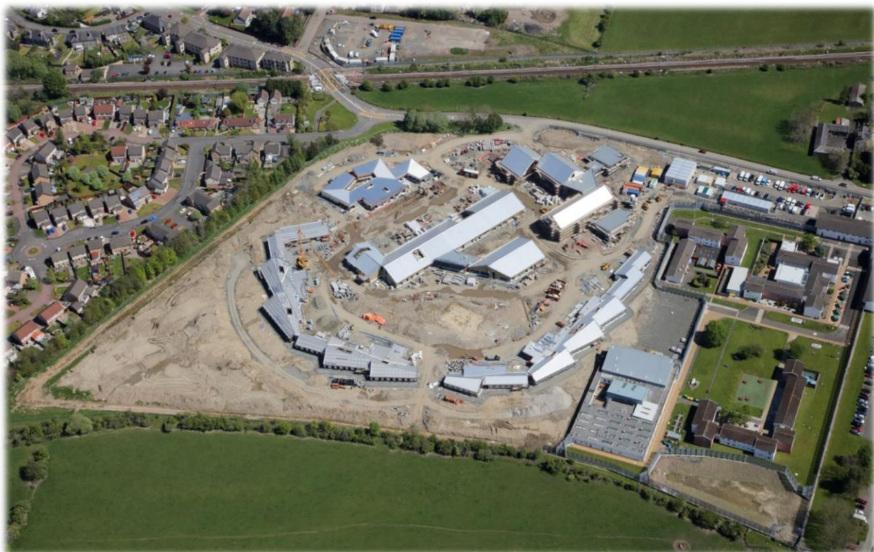
Women's National Facility, progress at March 2021
