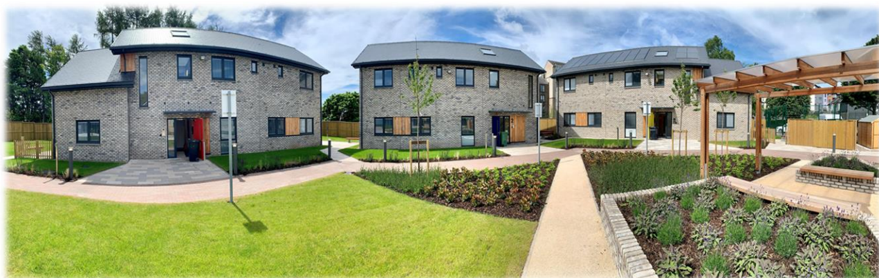
External view of the new Community Custody Unit (CCU) Bella in Dundee
